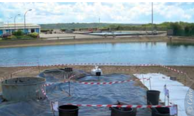
Decontamination and waste areas.
