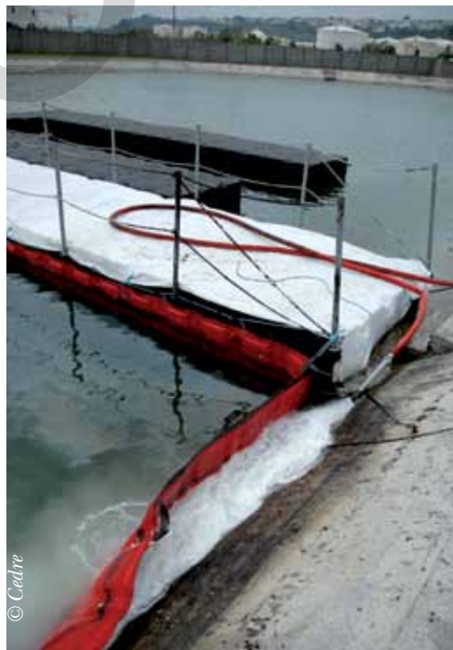
Protecting a floating pontoon using geotextile
