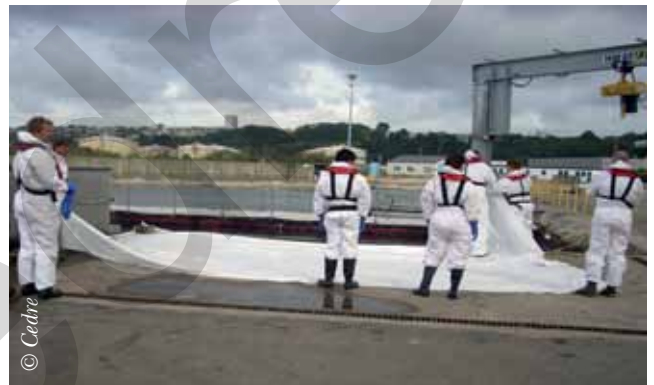
Protecting the quay with geotextile
