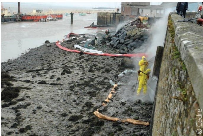
Pressure washing a wall and riprap
