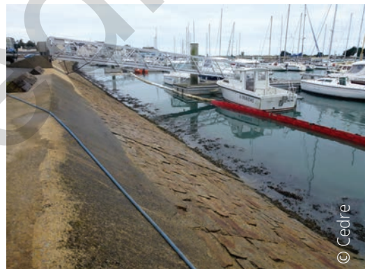
Oiled quay and containment using booms
