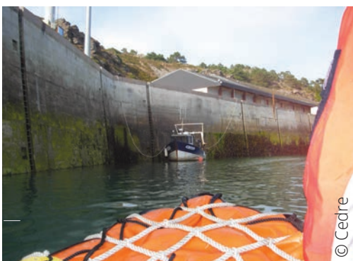
Boat-based survey along a quay wall
