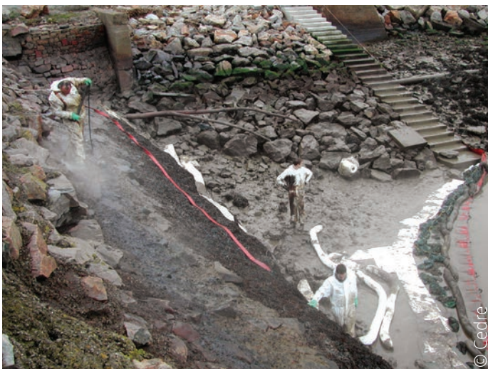
Recovering washing effluents using sorbent pads, pompons and booms
