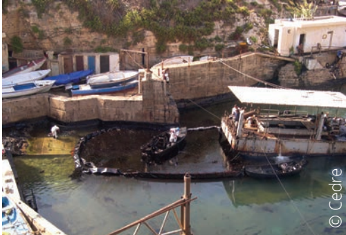
Pumping oil and storing it onboard a barge
