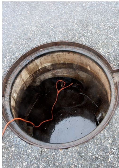
Plugging a manhole
