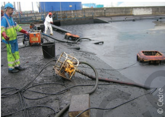
Recovering oil from a slipway with an oleophilic skimmer
