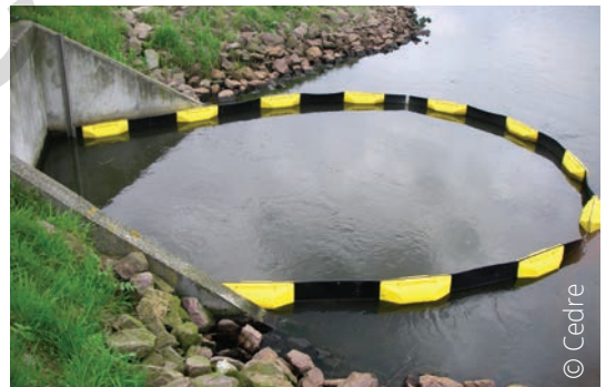
A permanent boom installed at an outfall
