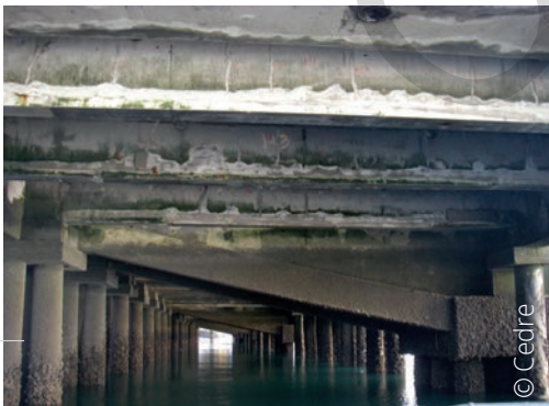
Boat-based survey under a piled wharf
