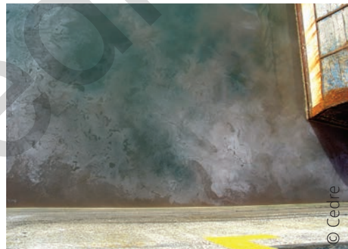
Scattered release of organic matter (fish processing wastewater)
