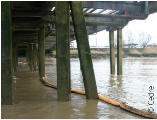
Sorbent boom below a wharf
