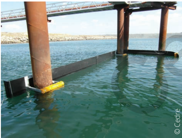
Permanent boom attached to a wharf
