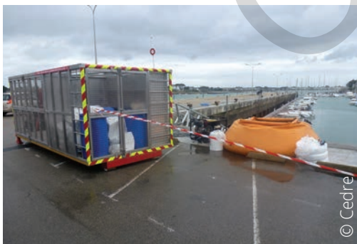
Logistics area adjacent to a clean-up site
