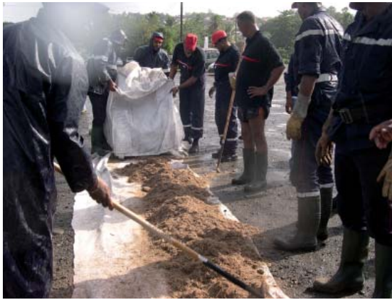
Building a makeshift boom: wire, geotextile and bagasse
