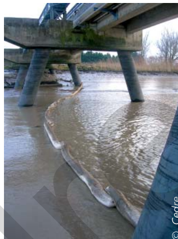
Booms (type E) to reduce the spreading and recover the oil on the Garonne
