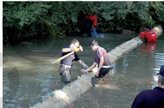
Installing a straw dam on a river
