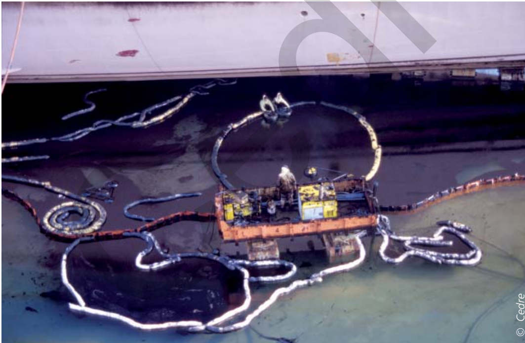
Operators containing oil around a skimmer using sorbent booms
