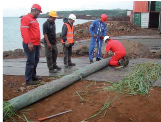
Makeshift boom surrounded by wire
