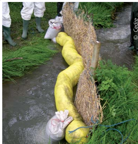
Makeshift filtrating dam
