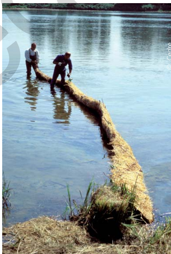
Installing a filtering dam made from straw, branches and wire
