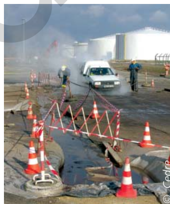
Pads (type B) used on decontamination areas
