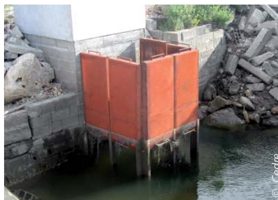
Filtration system around a water intake (3 rd level of protection)
