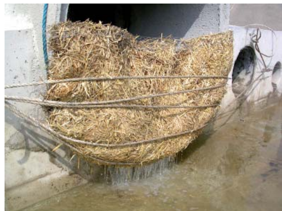
Filtration system made of straw on an outflow pipe
