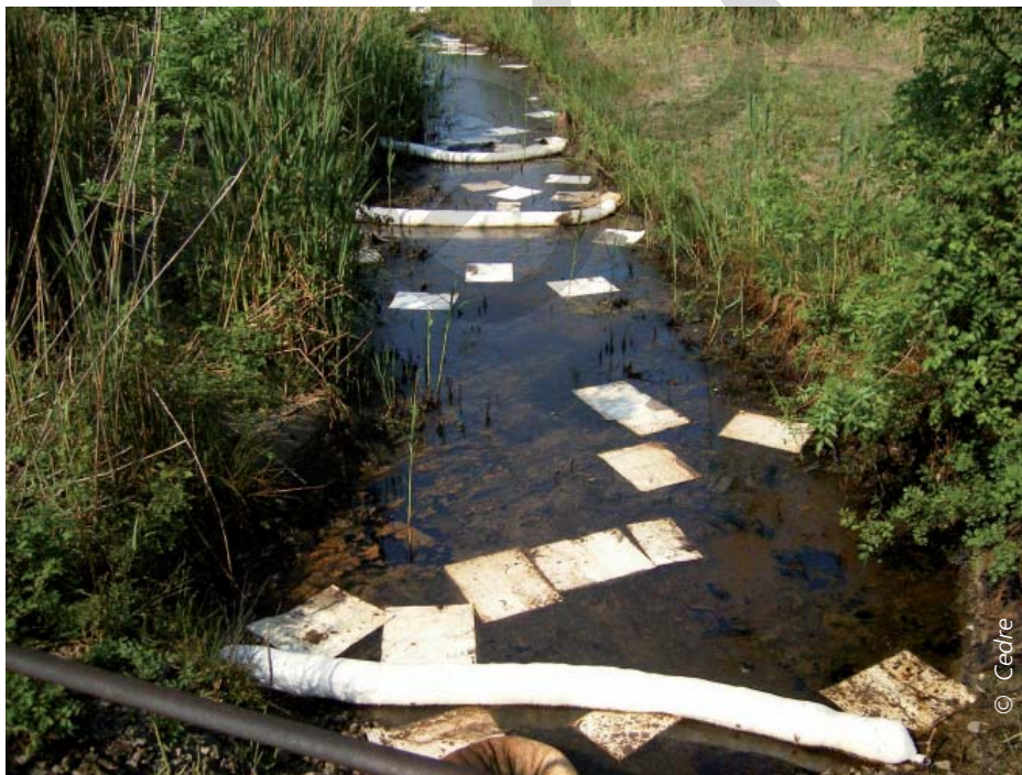
Sorbent pads and booms used to reduce spreading and recover the pollutant
