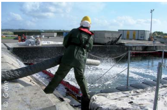
Applying sorbent using a blower
