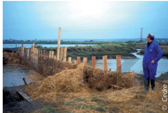
Filtrating dam made of straw
