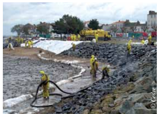
Mechanical clean-up on riprap
