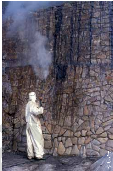
Pressure washing of a wall by a specialised cleaning company
