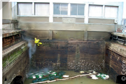
Clean-up operation conducted by a rope access technician
