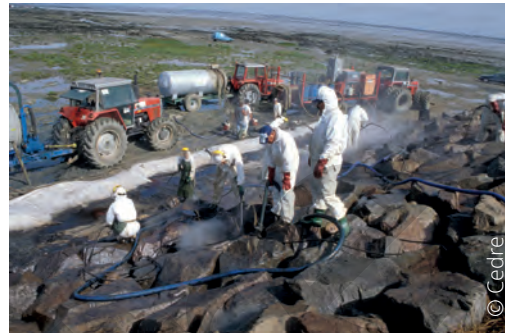
Mechanical clean-up operation
