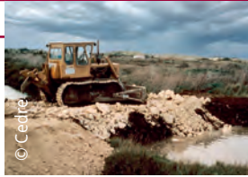
Rockfill dam without openings
