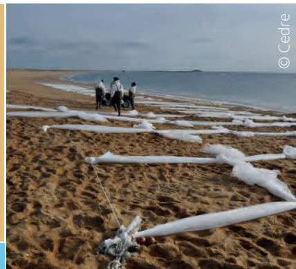
Rows of mop nets prepared at low tide for a surfwashing* operation at the next ebb tide
