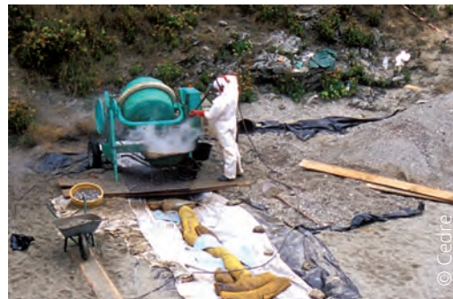
Washing in a concrete mixer
