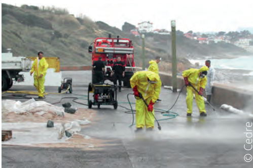
High pressure hot water washing
