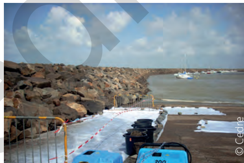
Preparing an access path to the clean-up site
