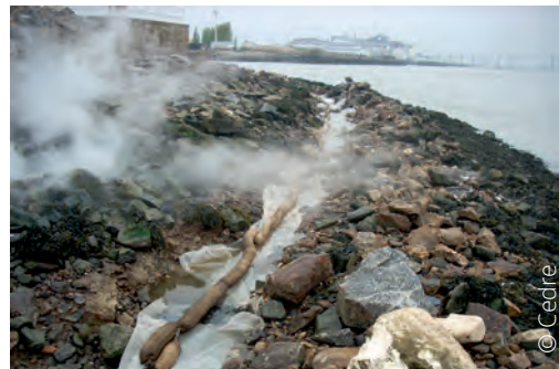
Recovering washing effluents from riprap
