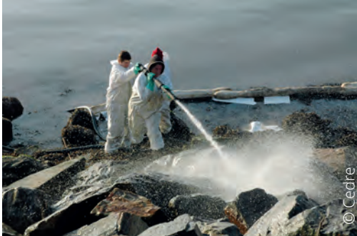
Flushing* operation on riprap
