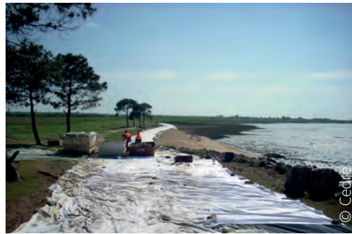
Ground protection and marking out vehicle tracks
