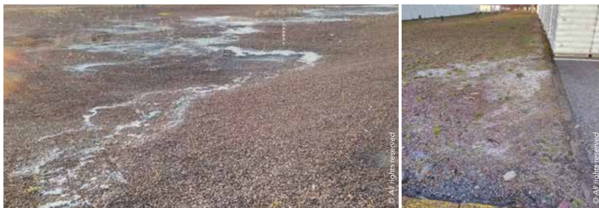
Figure 20. Plastic pellets on the ground in areas that are difficult to clean (old, deteriorated surfacing material and presence of vegetation) and where pre-existing pollution is present.
