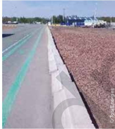
Examples of containment (netting, concrete kerb, flaps)
