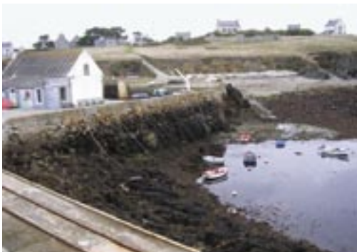
2. Manmade structures (ESI 8)
