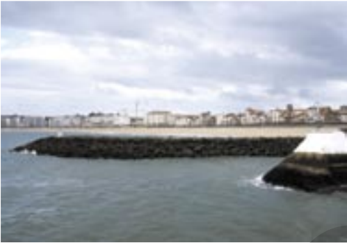
3. Manmade structure (ESI 2)
