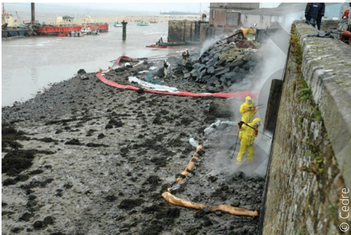
Pressure washing a wall and riprap
