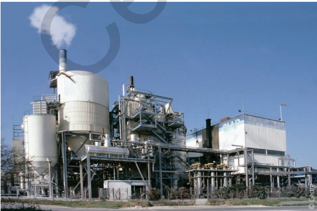
Hazardous waste treatment plant
