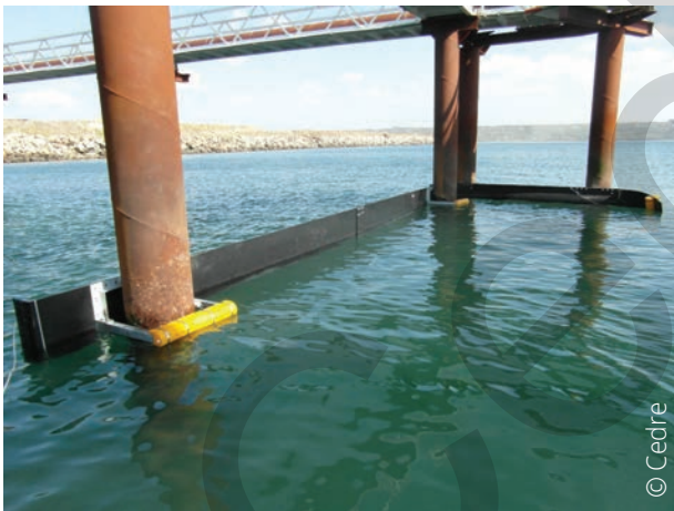
Permanent boom attached to a wharf
