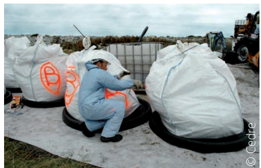
Labelling bags of waste prior to evacuation
