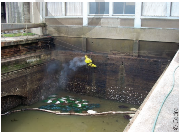
A rope access technician cleaning walls, recovery of washing effluents with sorbents
