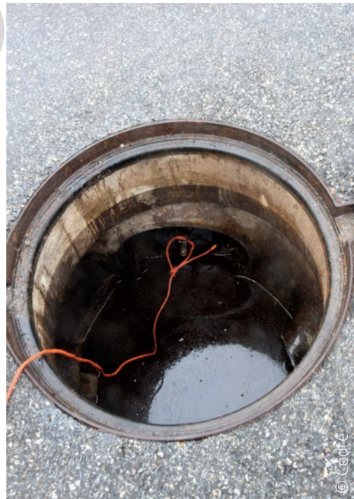
Plugging a manhole
