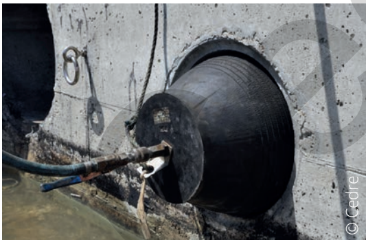
Using an inflatable plug
