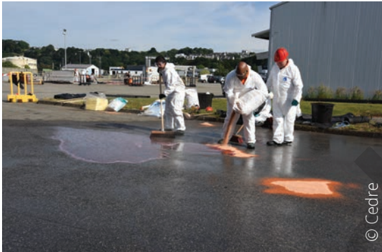
Applying bulk sorbents
