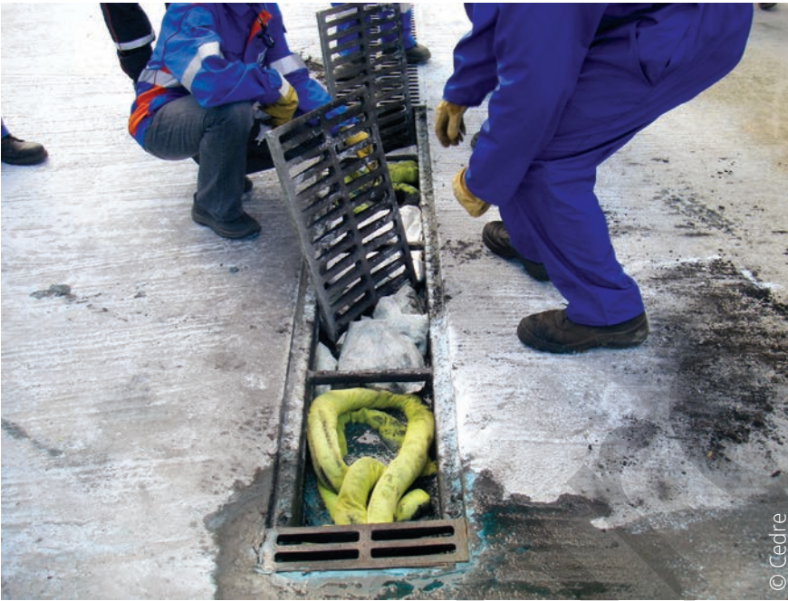
Packing a drain with sorbents
